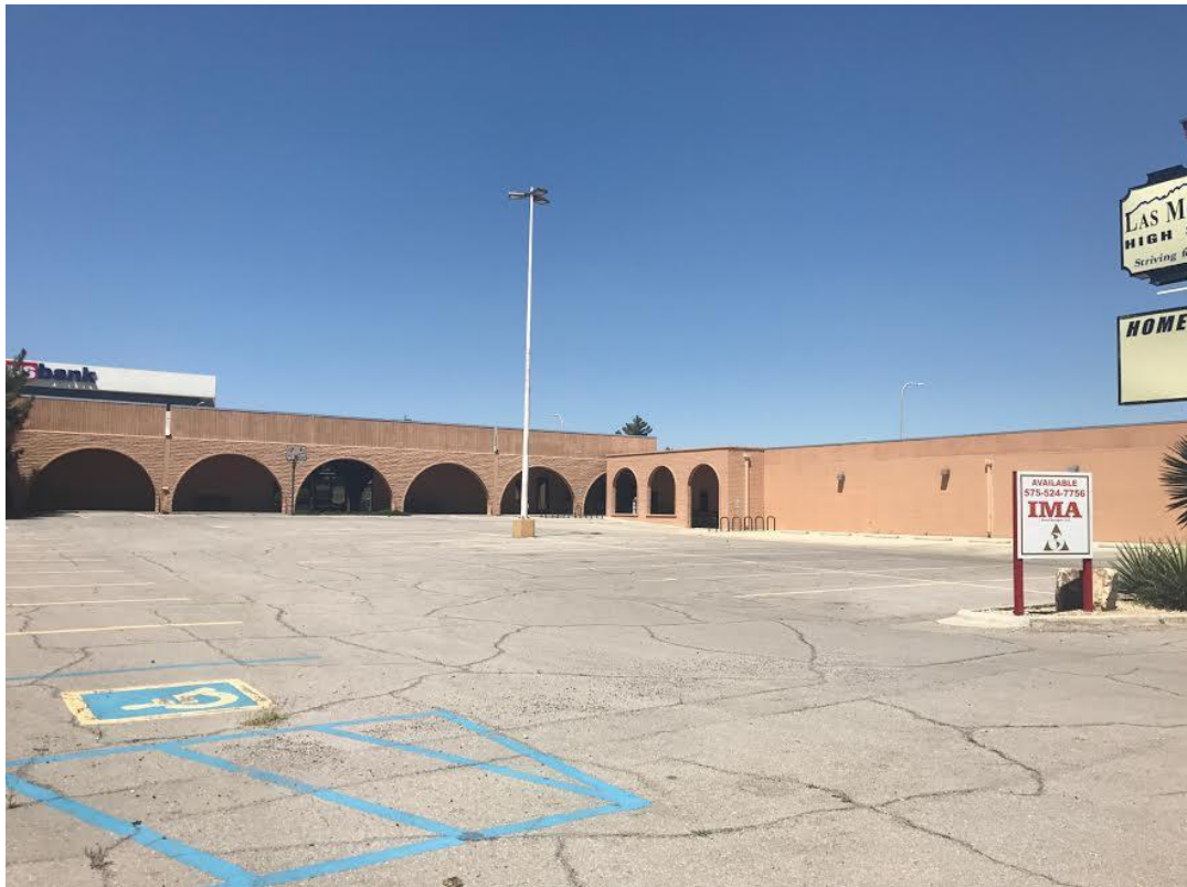
Appendix C, 201 E. Lohman facility image.
