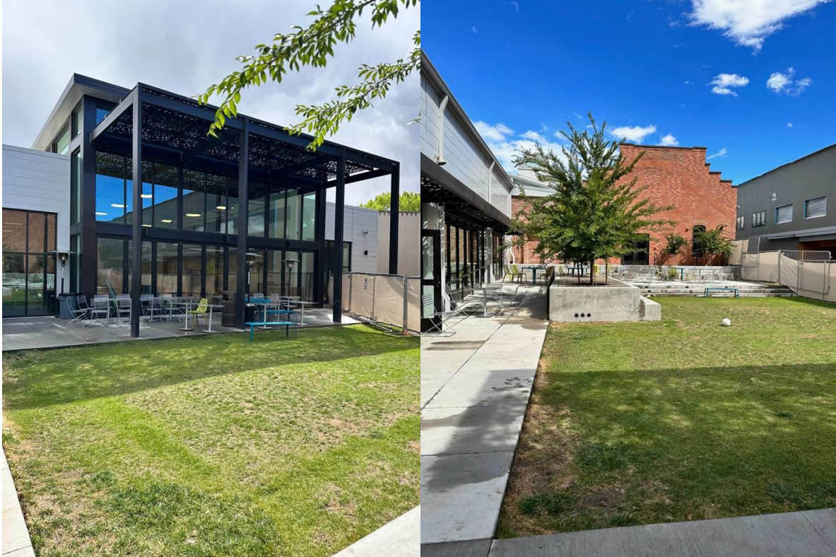
Courtyard, adjacent to cafeteria and new dormitory construction:
