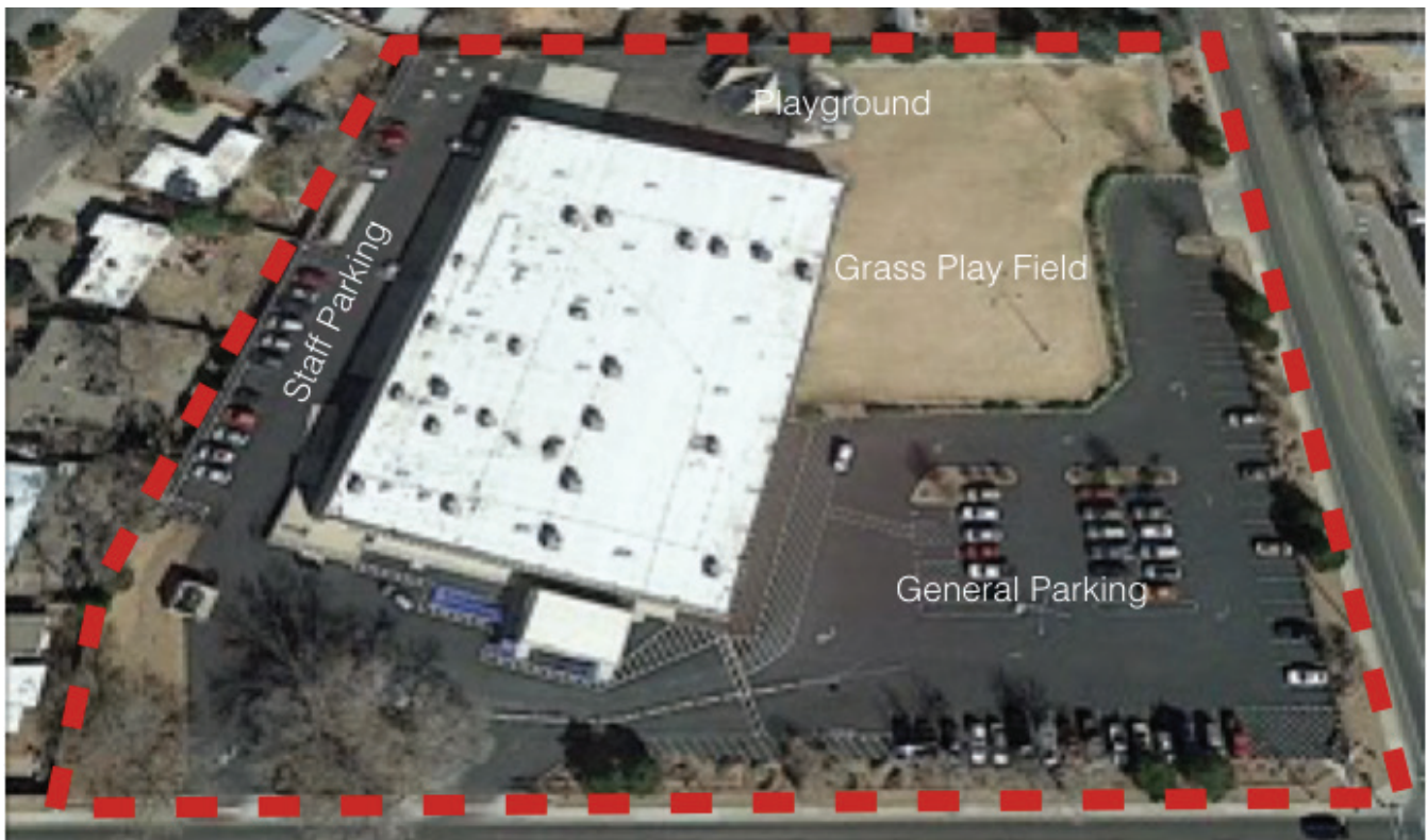
Exhibit 2-11 Aerial View of the SWLC Campus
