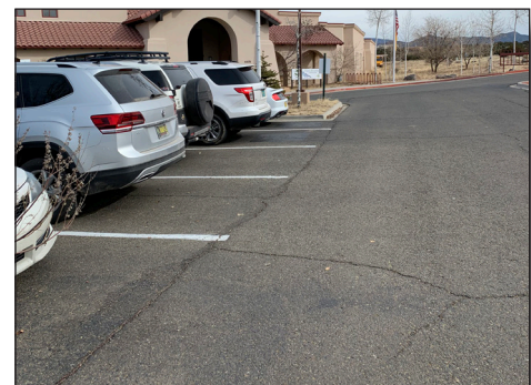
Parking lot areas also have a lot of asphalt cracks that need repairs and seal coat
