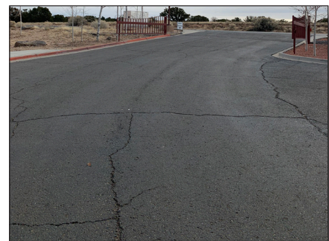
Southeast entrance to the site: multiple cracks in asphalt need repairs and seal coat
