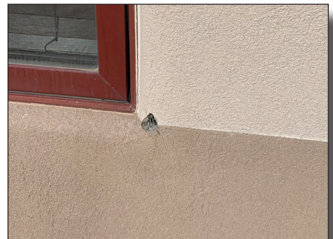
Damaged stucco along southside of building near Classroom #115
