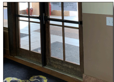
Repaint interior of main entry doors and install metal kick plates to protect from future damage
