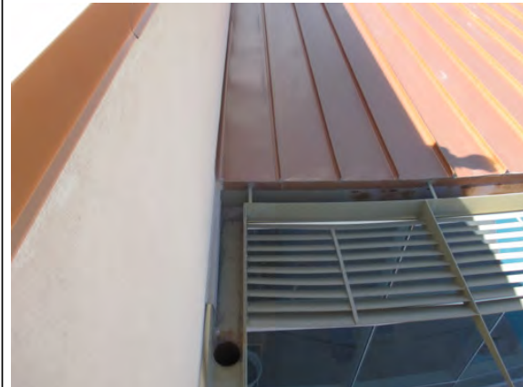
PHOTO #28- Entry curtainwall from above at corner where leak was reported
