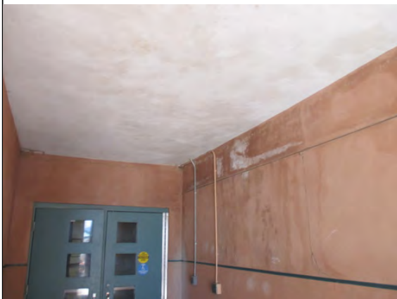
PHOTO #27- Hallway; evidence of leak at stucco
