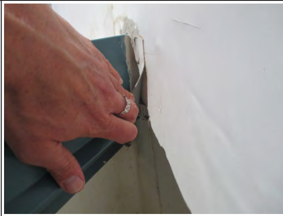
PHOTO #26- Roof membrane corner at parapet wall poorly sealed
