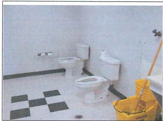
16. View of bathroom interior building 1
