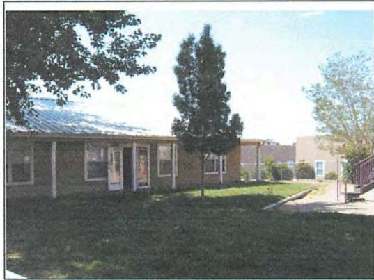
10. View NW of building 2 and playground area
