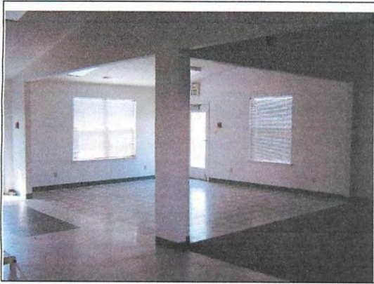
13. View of interior entrance area building 1. Note floor tiles and carpet.
