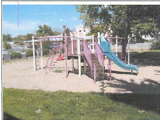
11. View NE of playground equipment E of building 2
