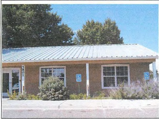
7. View N of S side building 1. Note metal roof.
