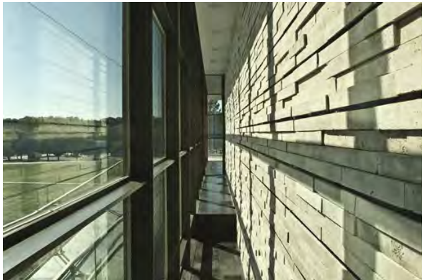
Attainable Home. Sunlight streams through windows to warm a stone wall. Attainable Home . 07 August 2023. www.greenbuildingadvisor.com/article/reassessing-passive-solar-design-principles
