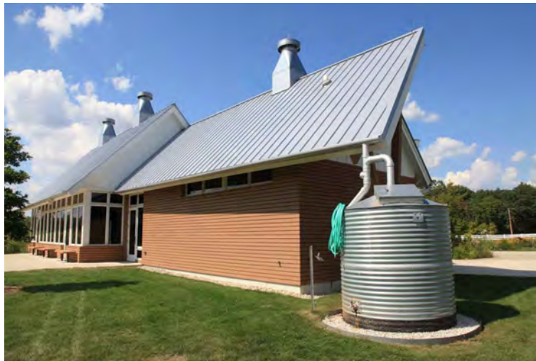
Vivify Roofing. Rainwater tank attached to a steep roof. Vivify Roofing . 07 August 2023. www.vivifyroofing.com.au/roof-restoration/roof-cleaning/colorbond-deterioration-rainwater-and-drinking-water/
