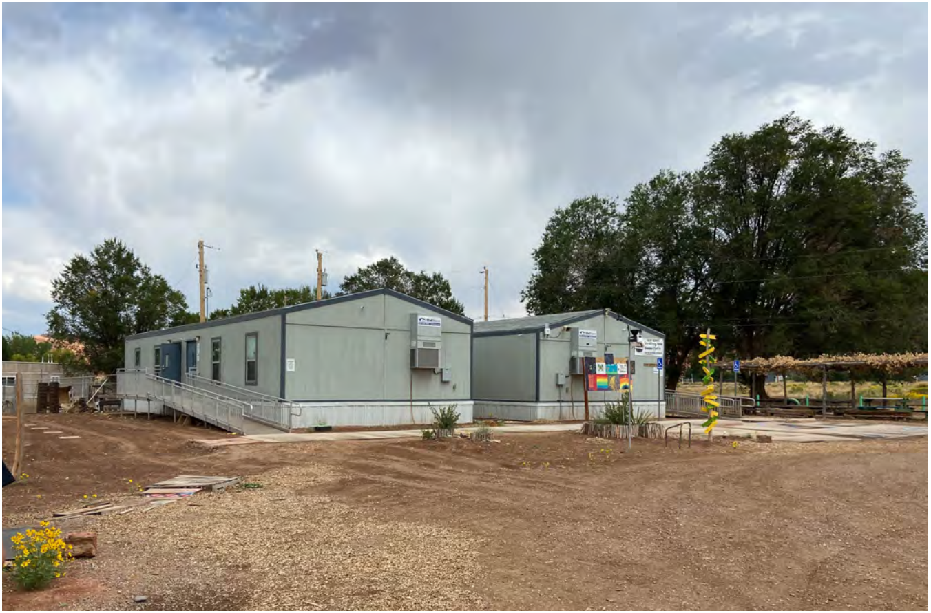
Existing Modular Classroom Buildings - Looking Northeast
