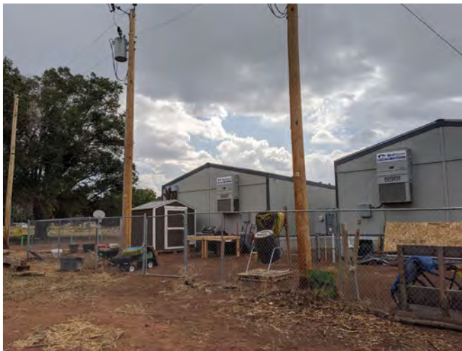
Figure 03: View of Current Portables
