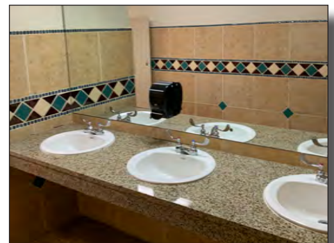
Typical student restrooms: ADA compliant
