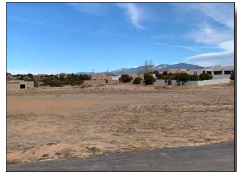
Outdoor playfield area on east side of building: no site fencing to secure campus
