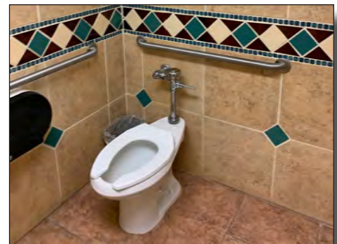
Typical student restrooms: ADA compliant
