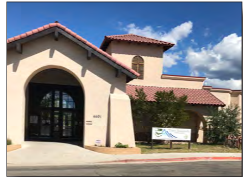
Main Entry to the School: Curbs need repainting
